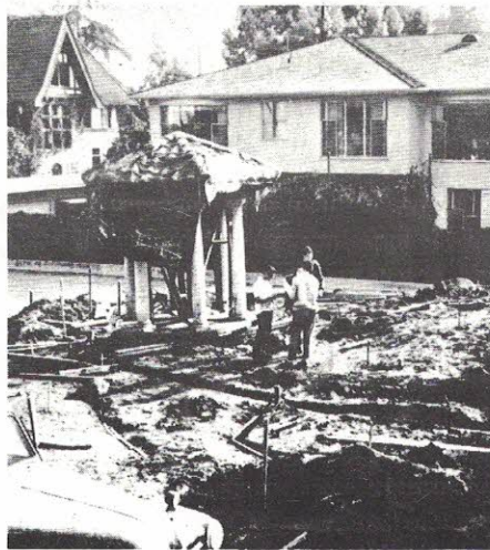
Work on new stream.
